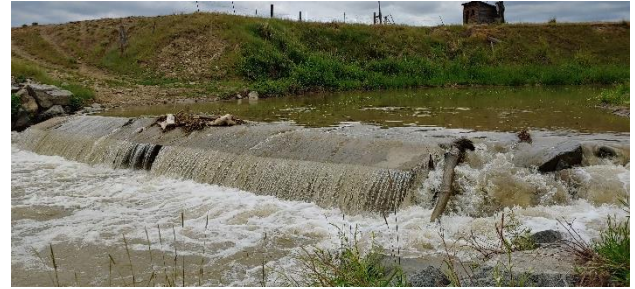
Photos are of the same crossing at low water (left) and during the irrigation season (right). Flows over run and erode such crossings, as well as running around the ends over banks.
