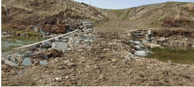
Photos are of the same crossing at low water (left) and during the irrigation season (right). Flows over run and erode such crossings, as well as running around the ends over banks.
